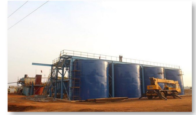
Expanded tank field being completed
