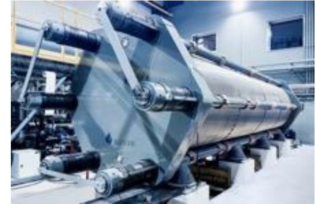
Sunfire’s alkaline electrolyzer installed at the MPREIS food center in Völs, Austria
